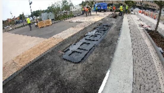
IN-ROAD CHARGING SYSTEM MADE OF UNDER-ROAD COIL SEGMENTS
