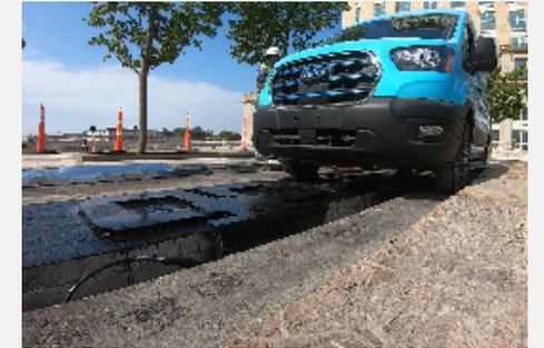
ENERGY TRANSFER USES RESONANT INDUCTION BETWEEN TWO COILS
